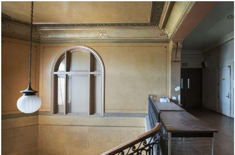
Central Stair at Second Floor
